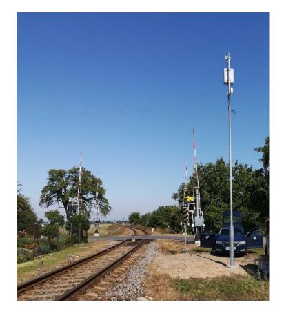
Pole with transmitters and antennas near the level crossing
