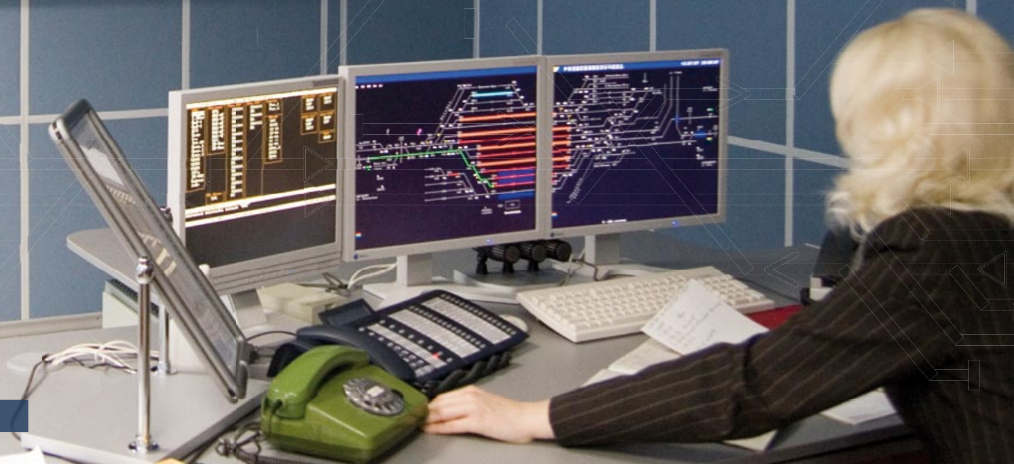
Dispatcher control place of the railway station Polock in Bielorrussia.
