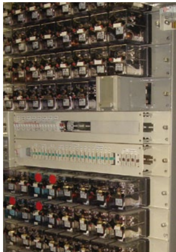
AHP-03 equipment complies with ČSN EN 50 125-3 requirements for installation inside the buildings without the climatic regulation.
