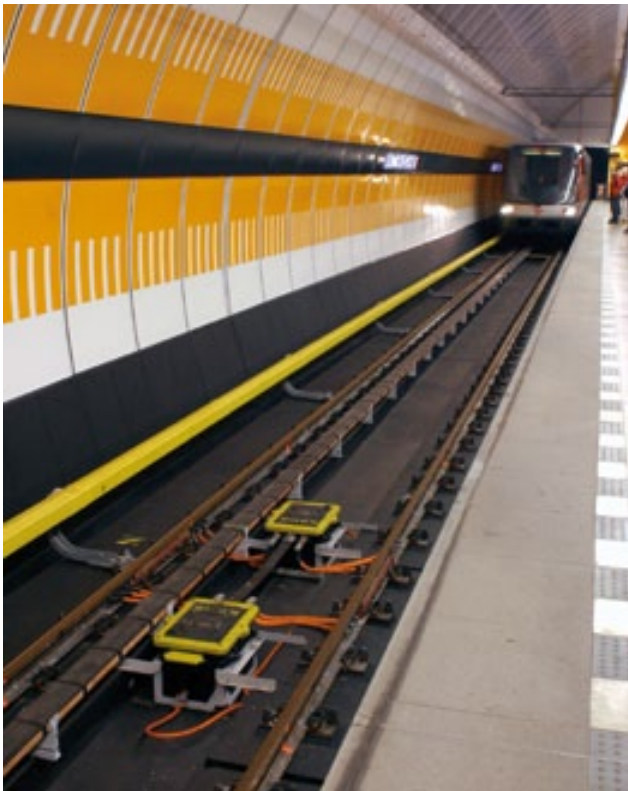
Impedance bonds at metro station railyard
