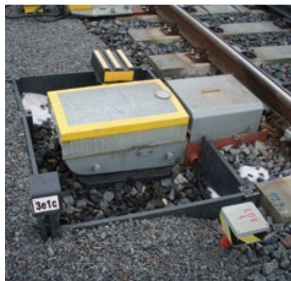
Flange fixation of point machine
