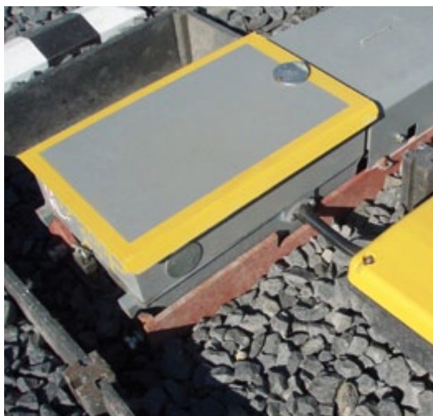
Configuration of point machine in hollow sleeper
