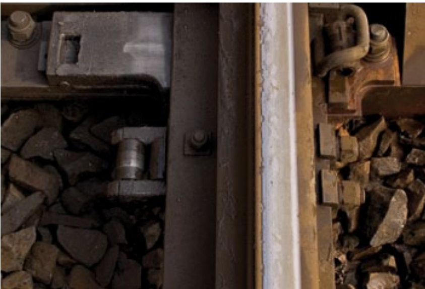
Lifting roller chair in close point blade position
