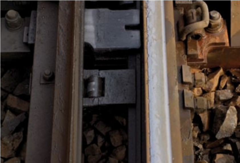
Lifting roller chair in open point blade position
