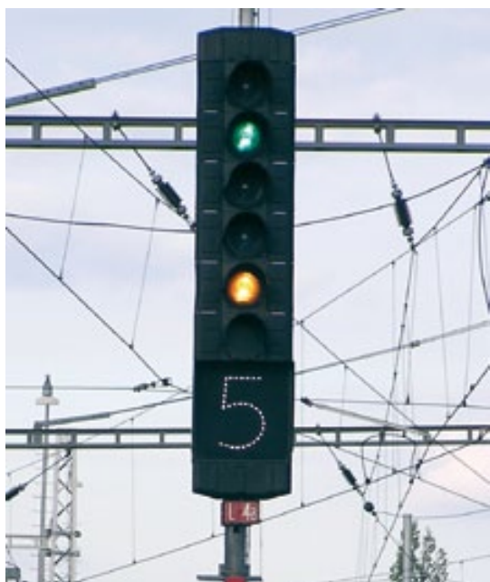
Example of signal lamps set
