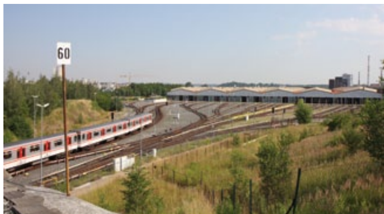
Metro depot railyard - ESA 11M+
